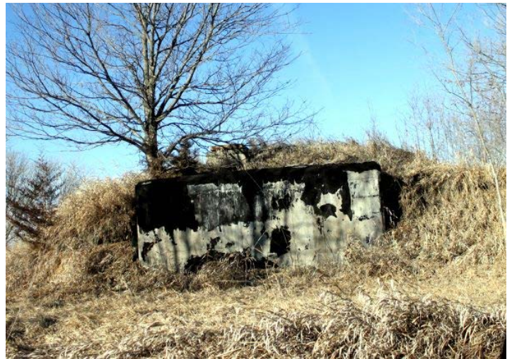
Back side of bunker
