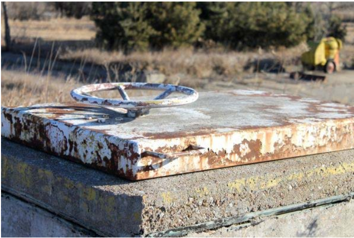
Escape hatch at top of bunker
